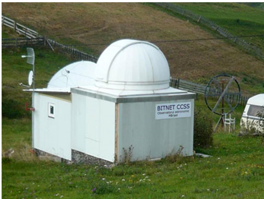
Fig.14. Our test infrastructure for satellite communication and surveillance of space experiments – in development. Located in Marisel, 1150 m altitude, 50 Km far from our offices in Cluj-Napoca. Electromagnetic quiet zone and without light pollution. The test bed hosts BITNET’s astronomical observatory and several antennas covering different radio bands, from few Hz to 13 GHz
