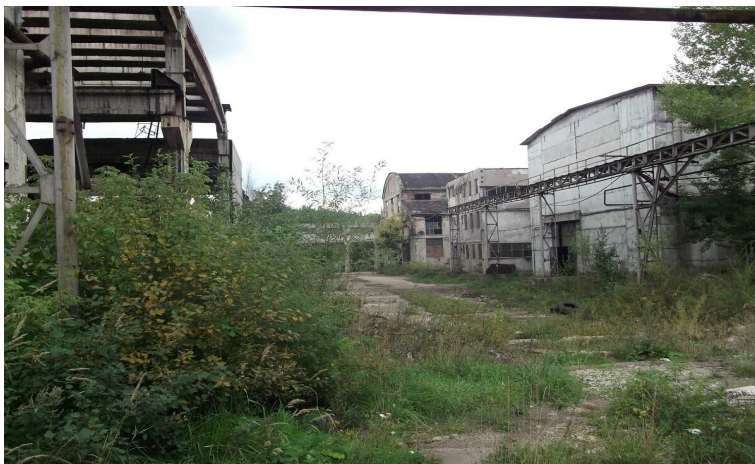
Fig. 4. Petroșani Central Workshops
