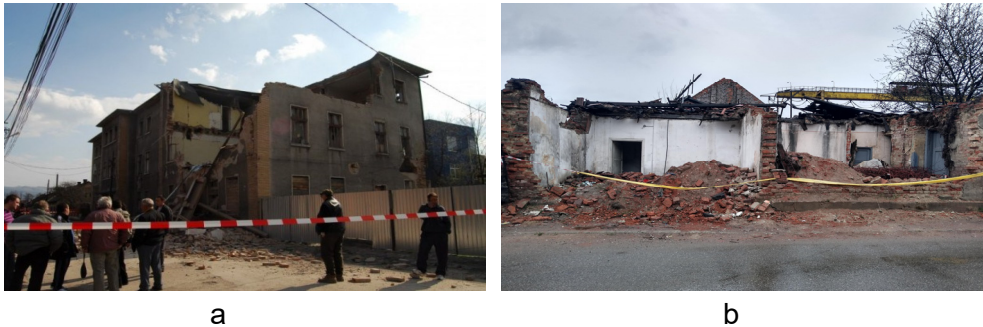
Fig. 5. CONSMIN buildings on Mihai Eminescu street (a) and Cărbunelui street (b)
