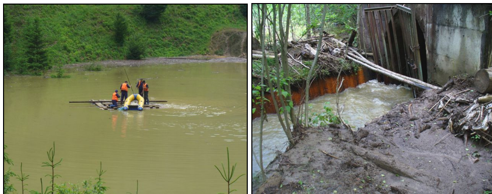
Fig. 4. Temporary lake formed in the top of the tailing dam endangering the downstream inhabitants and tourists located in Ostra village (detail of the diverting tunnel of the creek from the upstream area of the tailing dam, partially blocked with debris, and the operative measures of the emergency teams on a boat, for mitigation of the flood effects)
