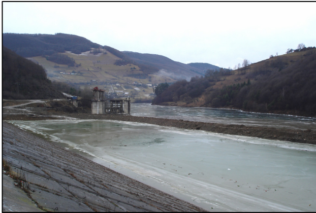
Fig. 3. Mihoiești reservoir during consolidation works for dam safety (Arieșul Mic)
