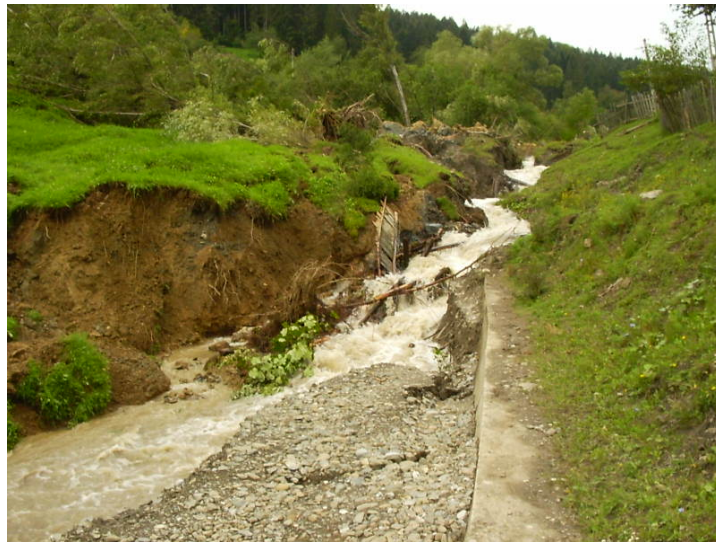
Fig. 3. Sometimes the reforestation is more feasible than other engineering works
