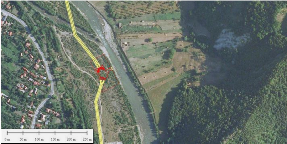
Figure 9. Small Hydropower Plant no. 1 and the surrounding area
