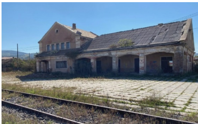
Fig. 5. Building of the station
