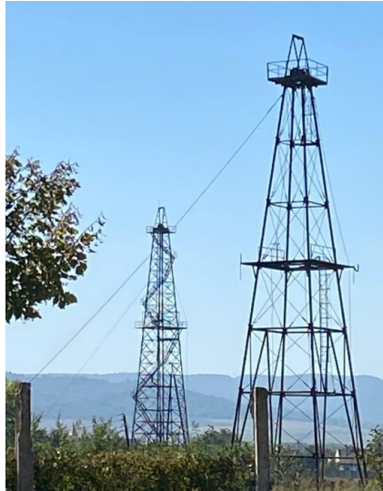
Fig. 3. The salt exploitation wells
