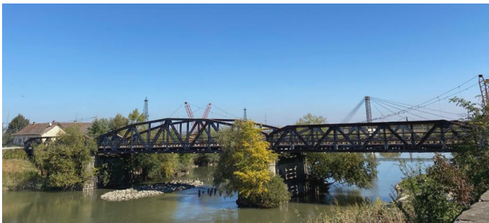
Fig. 4. The bridge over the Mureş River
