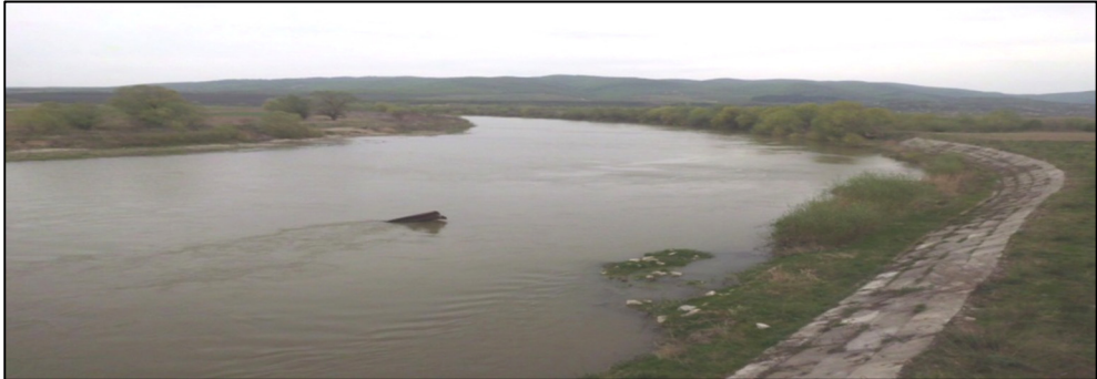
Fig. 11. Stabilization works of the left river bank at Ulmeni
