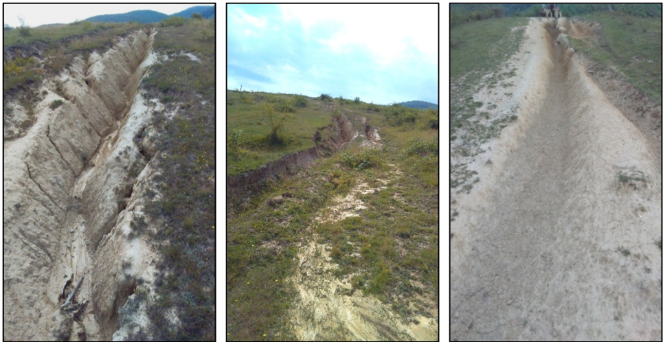
Fig. 6. Former dirt roads leading to the forest, affected by gullies
