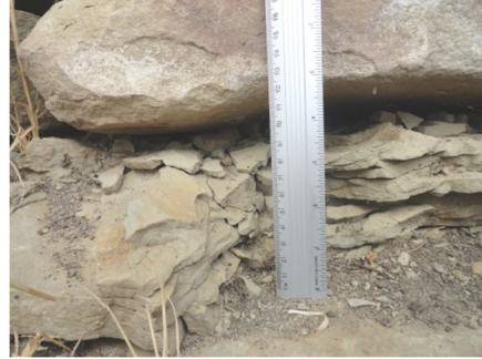
Fig. 3. Partial disintegration caused by severe delamination.
