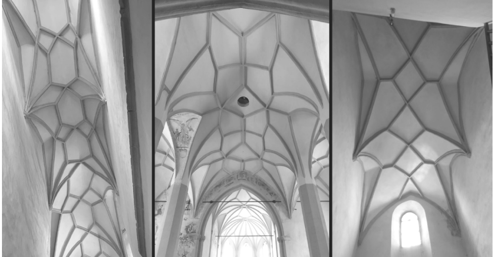
Fig. 1. The three different net vaults of the nave. (right: northern aisle, middle: main nave, left: southern aisle). Photos by Krisztina Fehér PhD
