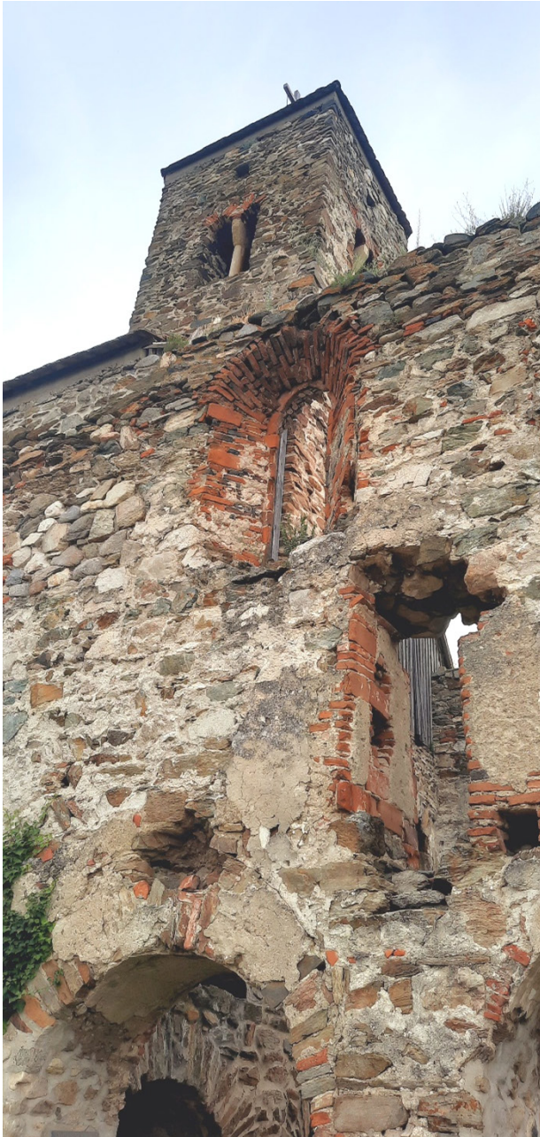
Fig. 10. Details of the consolidation with concrete beams, view from the south, 2023. (photo: I. Rus-Cacovean).
